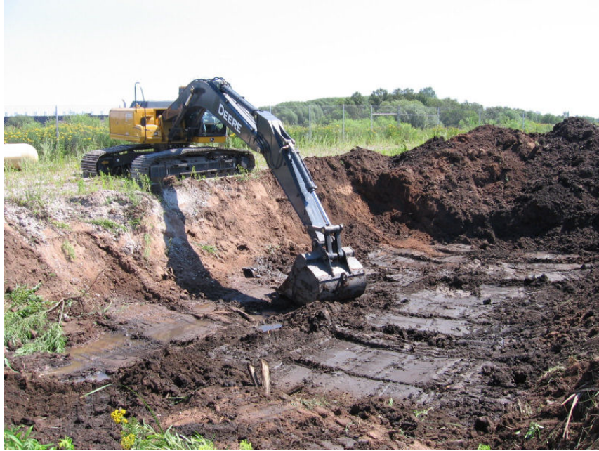
Figure 3. Preparation of the control cell prior to dike construction
