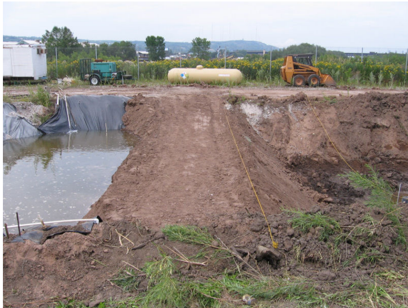
Figure 5. Completed dike and pool, with loader in the background (to the right of the propane tank).
