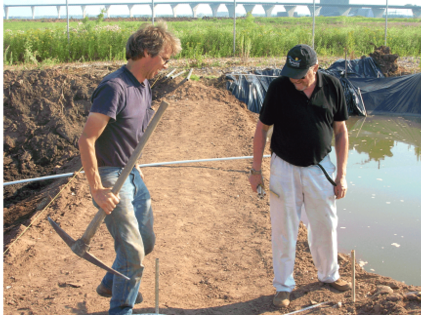
Figure 10. Dr. Doering and Larry Zanko on the completed dike.
