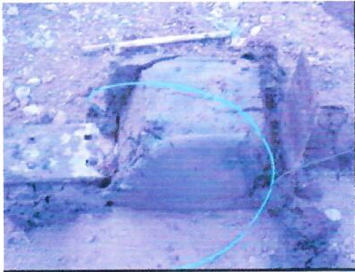
Figure 4 Material after Initial Removal
